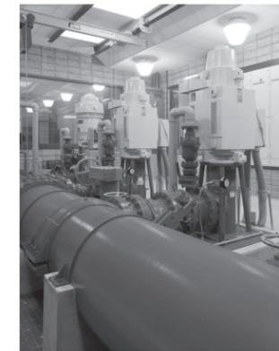
**Pictured above is the High Service Pump Room at the Water Filtration Plant. These pumps deliver drinking water to your community**
