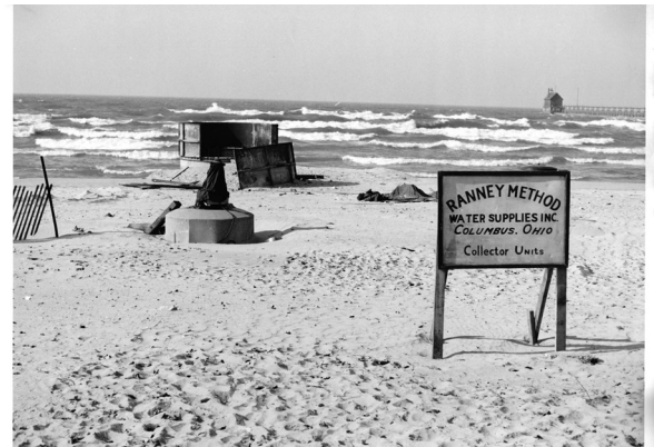
Pictured above is the City of Grand Haven's installation process of the retired 1950's Ranney Well Collectors (one of three). Designed to deliver 7 million gallons per day (MGD), but only could deliver 5 MGD. All three wells were removed in 2002.
